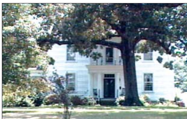
This mid-1800s farmhouse stands close to where the I-540 Outer Loop-Louisburg Road interchange is slated to be built.
